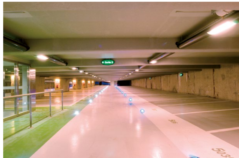
Parking Jean Jaurès, Avignon, France; lighting designer: Agence Hutinet, architect: Agence Lebunetel, photographer: Hervé Berthoule
